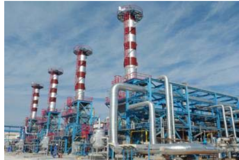
HP STEAM BOILER - LAVAN OIL REFINERY, IRAN
