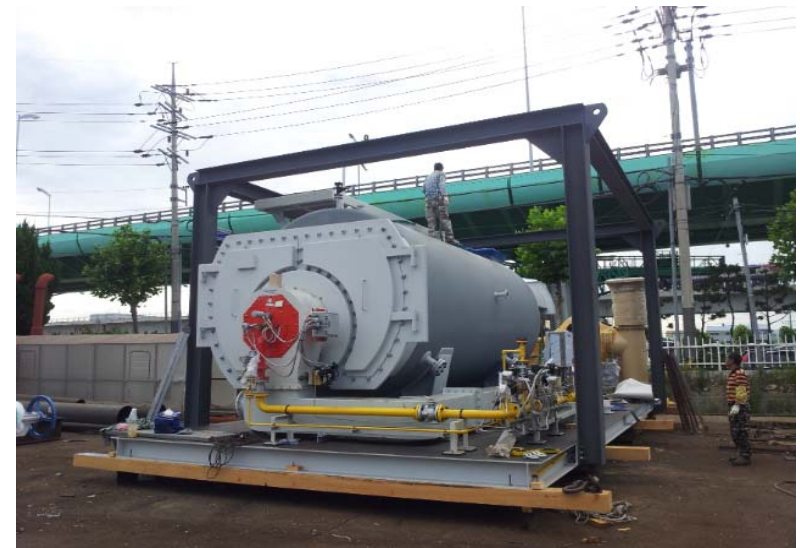
SMOKE TUBE BOILER - HYFLUX LTD, SIEMENS / TUASPRING, SINGAPORE
