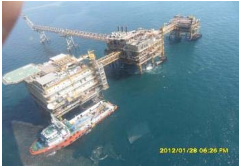
HASTELLOY HEAT EXCHANGERS ON PLATFORM - POGC, IGC / SP P1 REVAMPING, IRAN (TUBE-TO-TUBESHEET BY INTERNAL BORE WELDING)
